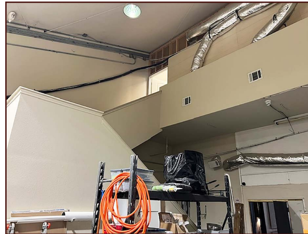
DOWN IN WAREHOUSE LOOKING UP TO MEZZANINE LEVEL
